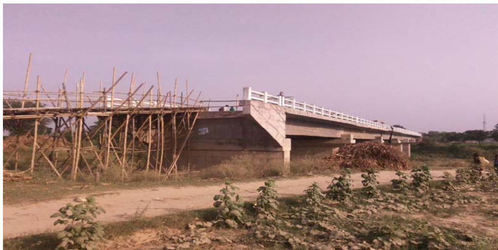
Incomplete bridge at Laluchak in Bhagalpur District
