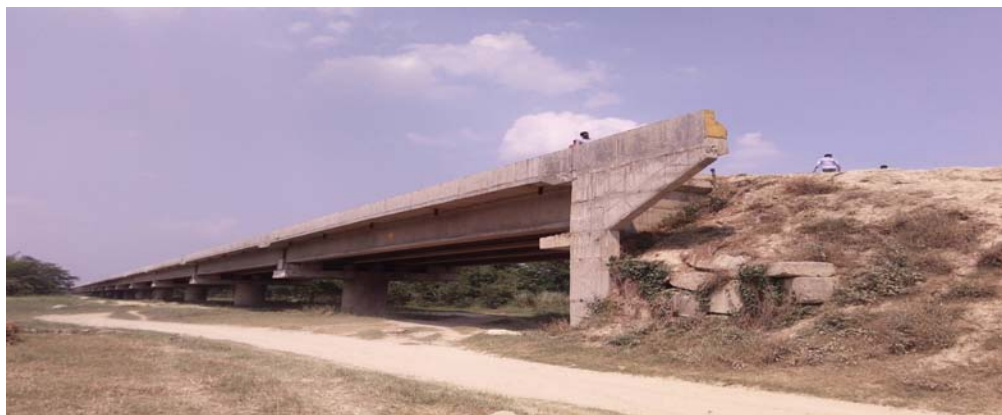
Incomplete bridge at Mandarghat in Sheohar District
