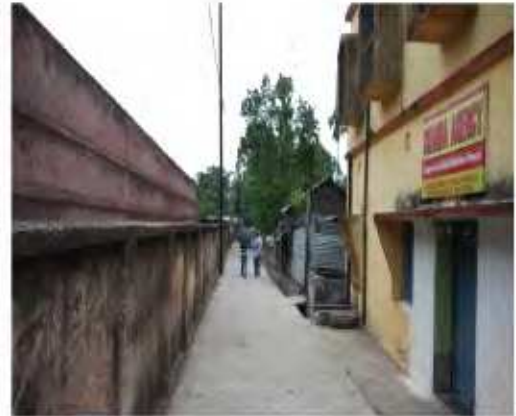
Private building in close vicinity to eastern perimeter wall of Raiganj DCH
