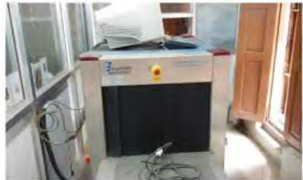
Defunct Baggage Scanner at Jalpaiguri CCH (June 2015)
