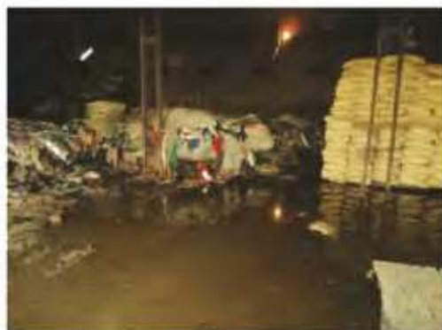
Water logging inside the godown at Taratala I centre
