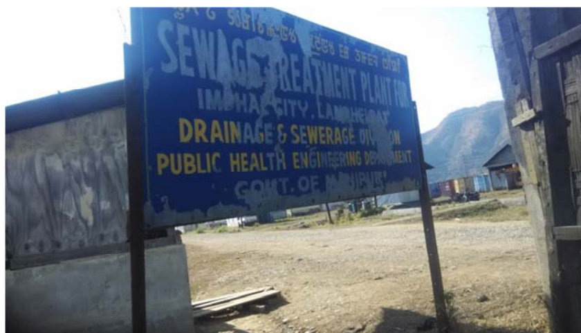
Sewage treatment plant at Lamphel
