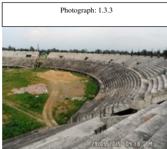
Construction of Gallery at the Main Athletic Stadium at MDSC, Dimapur.
