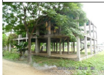
Construction of community centre at Chumukedima at a cost of ₹ 1.56 crore
