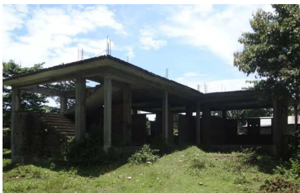
Construction of a Tribal Rest House at Barpeta town (8 July 2015)
