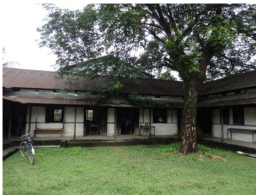
Dilapidated building of ITI Srikona (18 June 2015)
