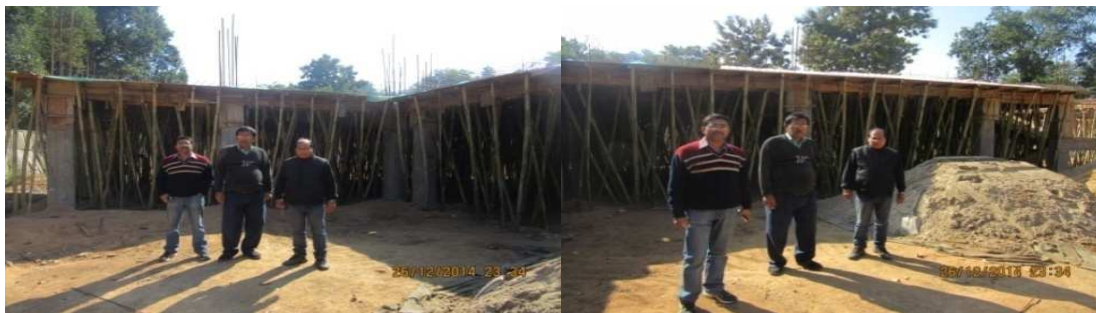
Construction site of guest house at Children Park near Kohora Range Office (26 December 2014)
