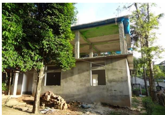
Construction of Boys' Hostel at Narikal Basti, Guwahati (25 June 2015)
