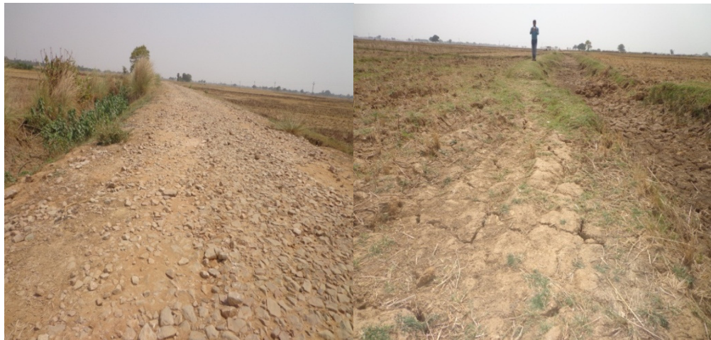
Constructed part of the road (0.85 km)
