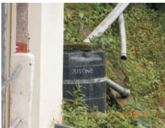
Tank to collect effluents at Kulikawn Hospital
