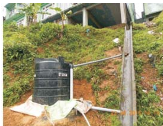
Tank to collect effluents at State Referral Hospital, Falkawn
