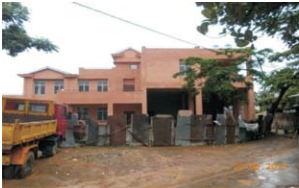
Fire and Emergency Building at ITI Aizawl Land
