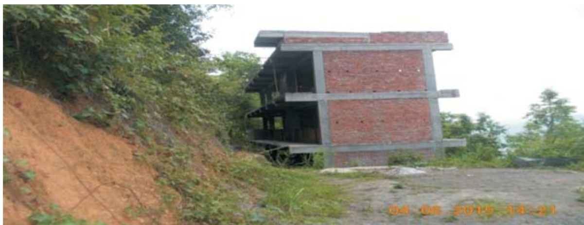
Site of abandoned boys hostel construction at ITI, Saiha
