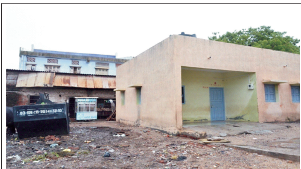
Picture 6 : AC near garbage containers at Daru Khota, Khambhat NP
