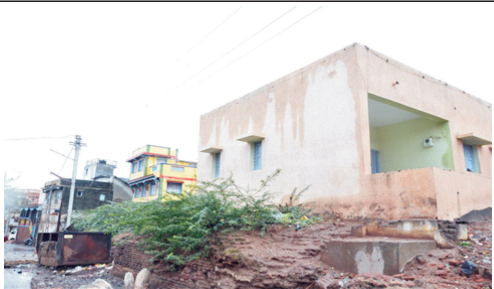
Picture 5 : AC near garbage containers at Khari Vadi, Khambhat NP
