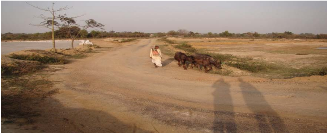
Picture 3: Road under Gramin Sadak Yojana of Rural Works Department, GoJ passing through ash pond area of KTPS
