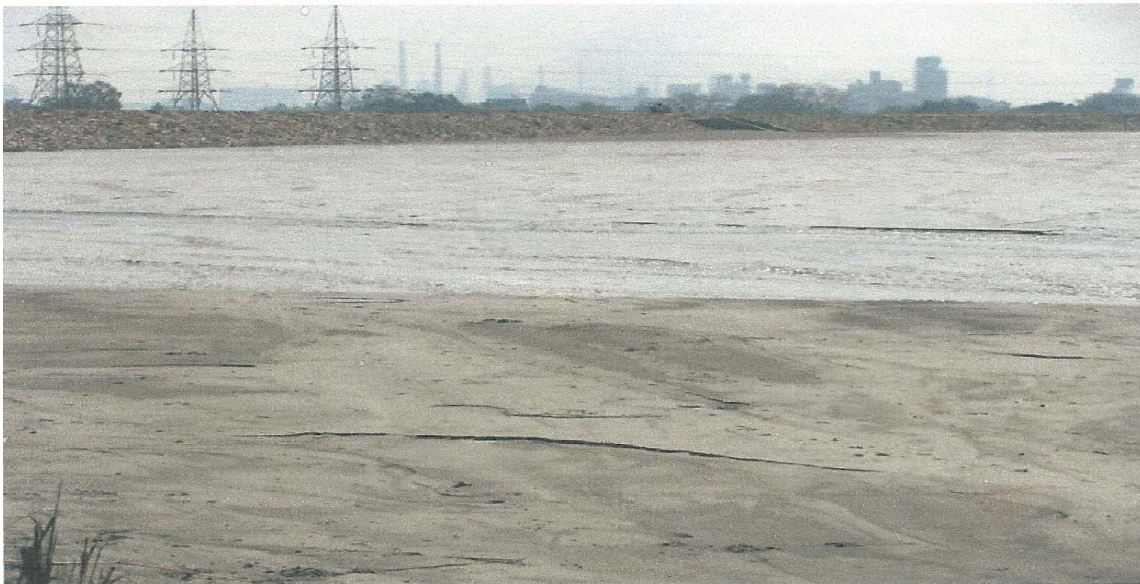
Picture 2: Filled up Lower capacity lagoon of Ash Pond – DSTPS
