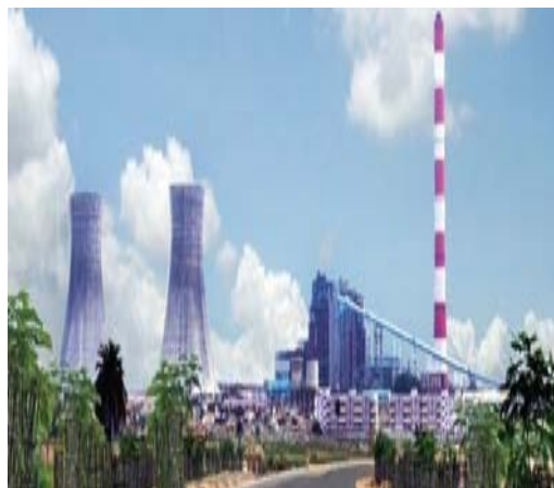
Picture: 1 Power plant
