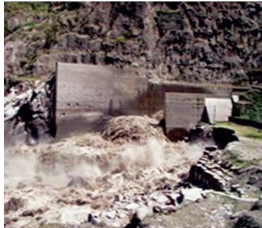
Flood water discharge form Radial Gate
