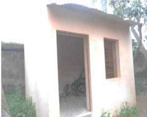
Photo 17: Cooking of MDM was not done in the newly constructed kitchen shed due to small size(10'X9')
