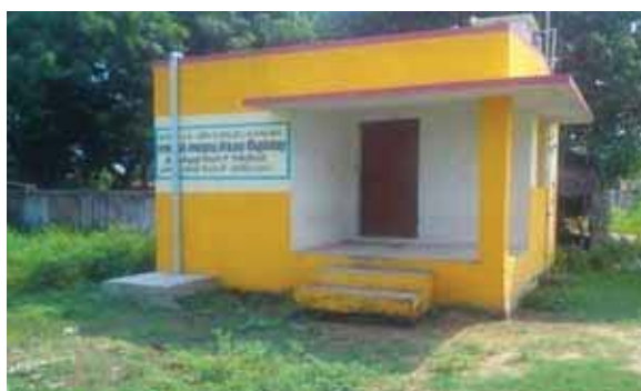
Photo 15: KCS was not handed over by the contractor for 2 years as a result the constructed building was not used (PUMS, Pullarambakkam School)
