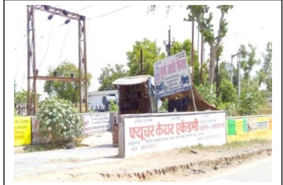
Unused Kudaghar and dhalao near power-house along the highway in NP-Bakewar, Etawah (27/06/2015)
