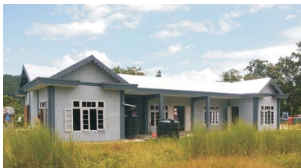
Pic 3: Unoccupied Lodge
