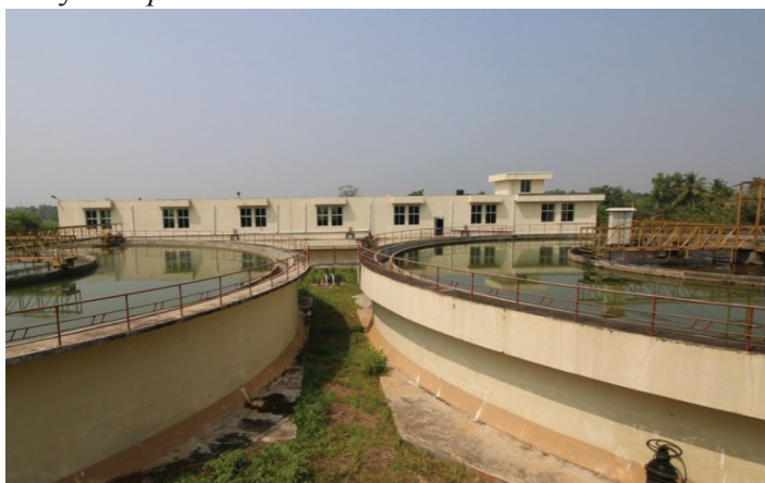
Completed water treatment plant remaining unutilised
