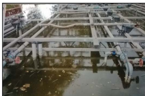
Growth of moss in the stagnated water of the computerised musical dancing fountain at Kuppanna Park, Mysuru (19.06.2014)
