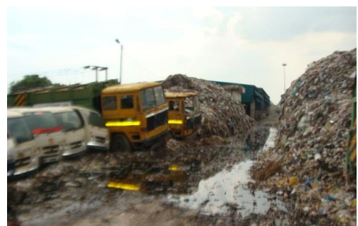
Non-operational MSW processing plant at NN Aligarh (24.07.15)
