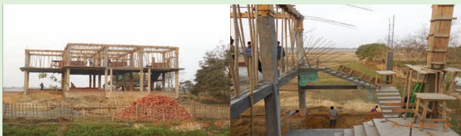
Wayside Amenity Centre, Numaligarh
