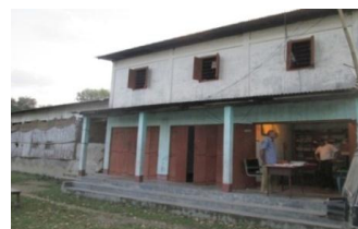
Bhakatpara PS operated from market shed (6 August 2014)
