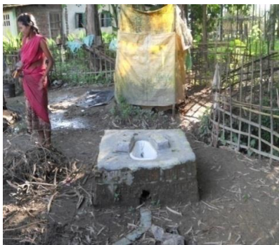
Toilet without superstructure at Rongpuria GP, Tinsukia (26 August 2014)
