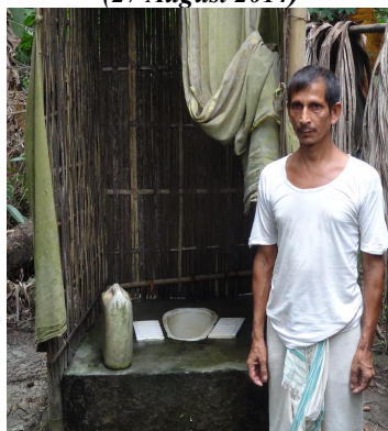
A toilet without door at Pub Bahjani GP, Nalbari (6 September 2014)
