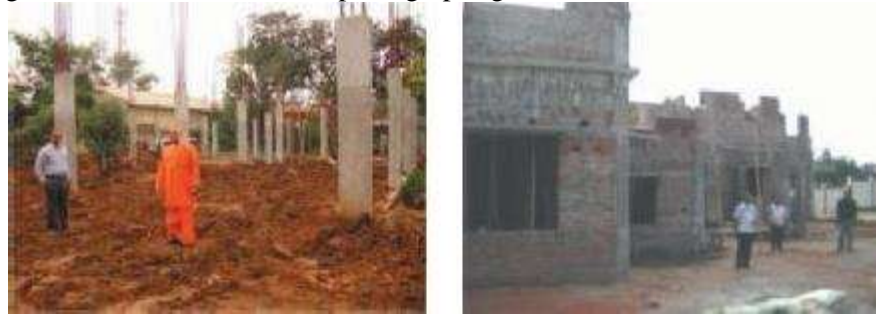
Partially completed hostels at Ranchi and Dumka
