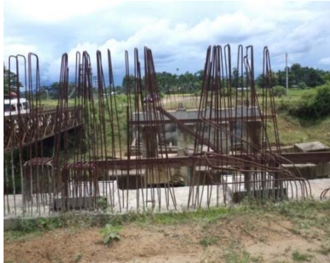
A. RCC Bridge at Rowa
