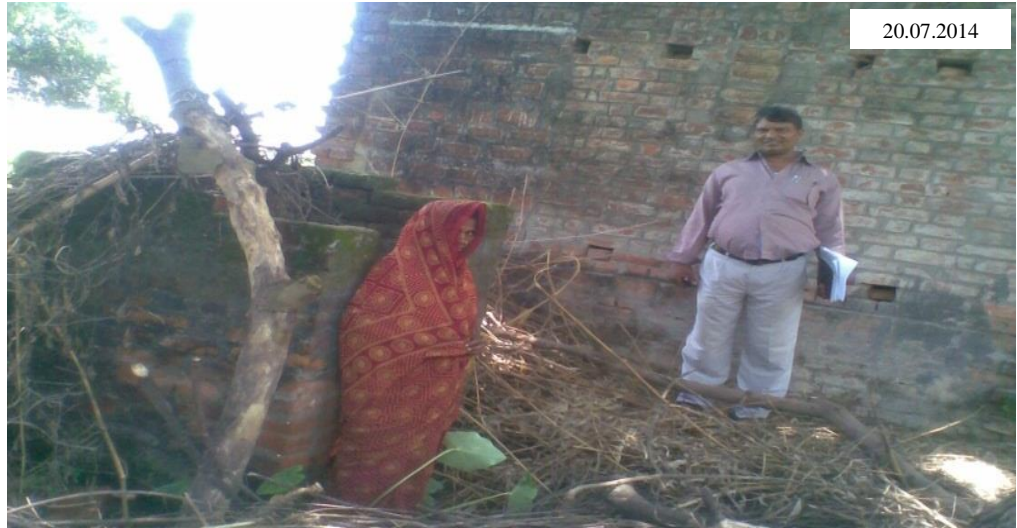
(Broken IHHL of a beneficiary of GP, Dhavarkan, block- Bhatpar Rani, Deoria)
