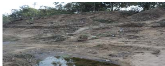
Embankment in Subarnarekha River not restored
