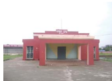
Renovation of Town Hall, Subarnapur
