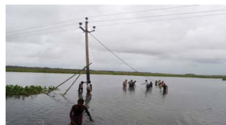
People in Puri working in water logged area to restore power supply
