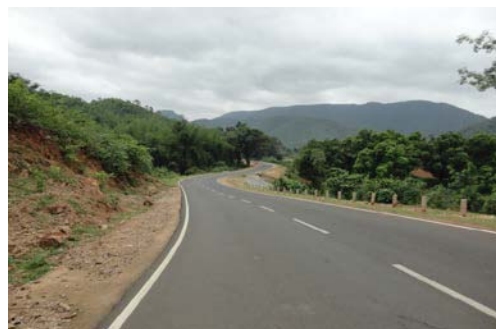
Completed stretch of South North Corridor
