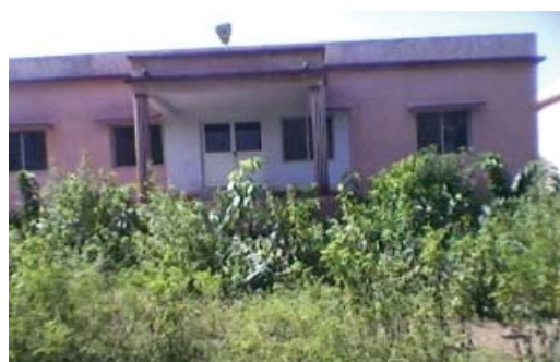
Non-functional CHC building at Boipariguda
