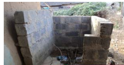
Latrine of a household of Kumelsingha GP of Bargarh district lying unused
