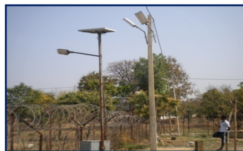
Installation of lighting system at Meghpal ANPP, Sambalpur without power supply
