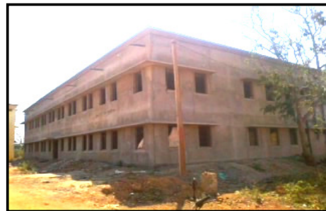
Construction of barrack at CPMF Headquarters, Koraput with RCC roof
