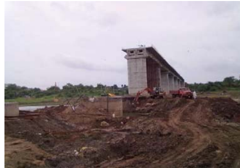
Photograph taken by Audit (27 June 2013)
