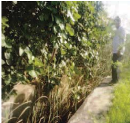
Thick vegetation and heavy siltation in canal
