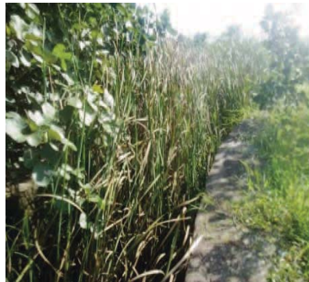
Thick vegetation and heavy siltation in canal
