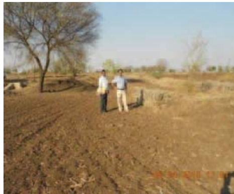
Field Channel on outlet left I of Minor 86 on Kukadi Left Bank Canal
