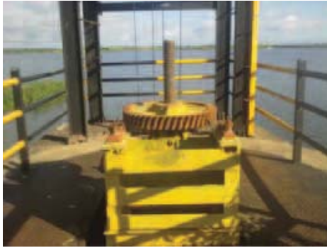
Absence of shaft rod and leakage of water in the canal in Jambnala project, Yavatmal
