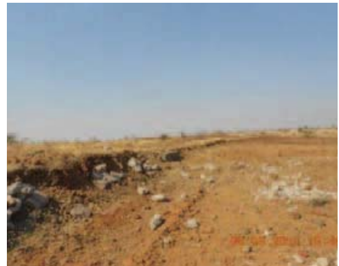
Field Channel on outlet right of Sub-minor 3 on Minor 90 of Kukadi Left Bank Canal
