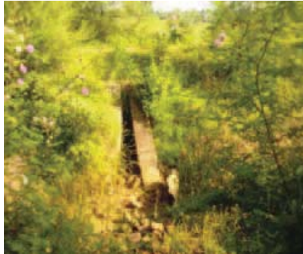
Broken outlet and non-functional structure
