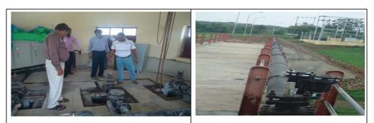
Intake well-cum-pump house and approach bridge to the intake well, installed pipe line, air valve and sluice valve installed at Village Velgipada, Sardarpur in Dhar district for covering 44 habitations in Badnawar/Sardarpur blocks of Dhar district for pumping raw water to the treatment plant, the work was completed in March 2013. After testing, water is being supplied since September 2013.
