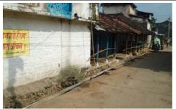
Over Head Tank constructed and GI pipeline can be seen layed at a cost of ₹ 6.50 lakh in October 2011 within village Ratanpur Girdhari, Raisen District from where household connection are provided. The PWSS is handed over to Mendki Panchayat of the village, having 115 individual household connections.
