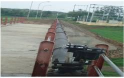
Intake well-cum-pump house and approach bridge to the intake well, installed pipe line, air valve and sluice valve installed at Village Velgipada, Sardarpur in Dhar district for covering 44 habitations in Badnawar/Sardarpur blocks of Dhar district for pumping raw water to the treatment plant, the work was completed in March 2013. After testing, water is being supplied since September 2013.
