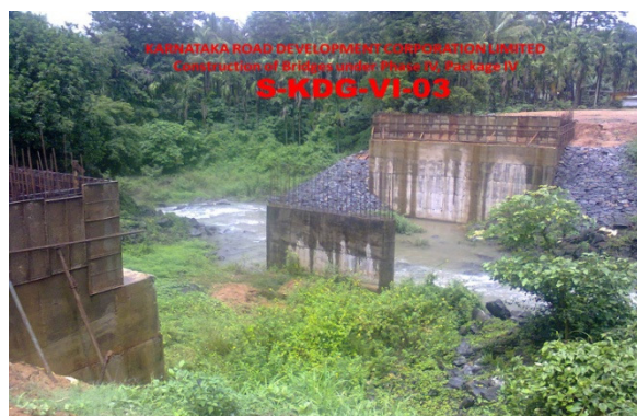
(Bridge on Madikeri-Kutta road across Lakshmantheertha river- photo dated May 2013)
