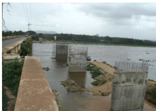
Bridge on Hosepet -Shimoga Road at Honnali (June 2013)
