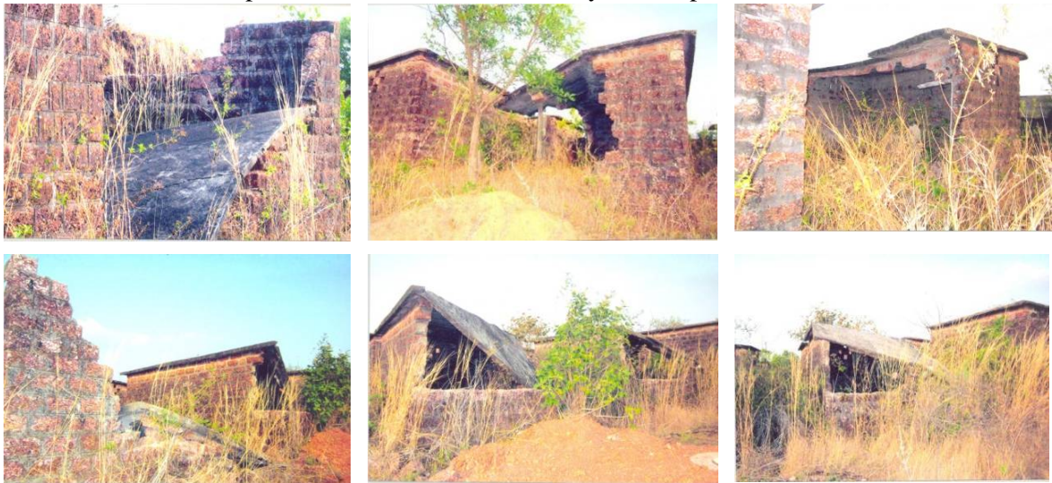
(Collapsed roofs and walls of Ashraya houses)
