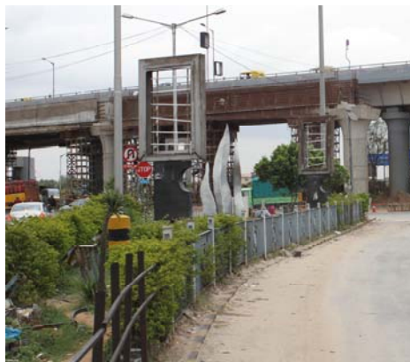
Damaged advertisement boards at Hebbal flyover
