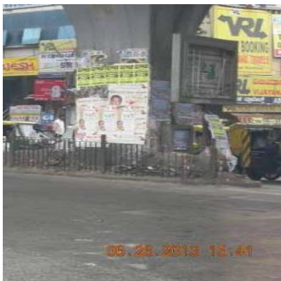
Damaged advertisement boards and posters pasted on the landscape of the Anandrao Circle flyover
