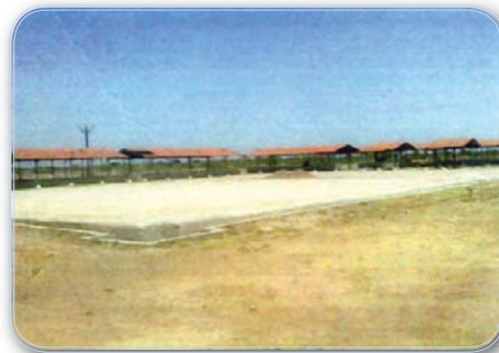
Picture 13 VCP at Thangadh, Surendranagar District (24.05.2013)
