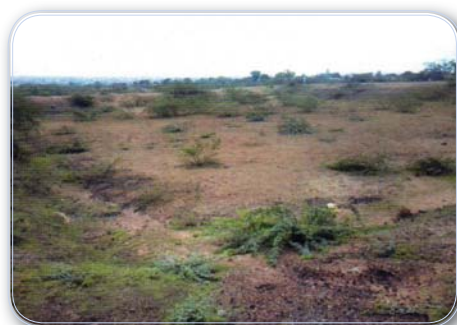
Picture 19 Incomplete SLF developed by GUDC, under GERRP at Bhachau, Kutch District (10.07.2013)
