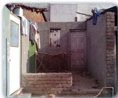
Picture 1 IAY house of Shaikh Rukhshanabibi Allahrakha, Village Moraj, Taluka Tarapur, District Anand (29.05.2013)
