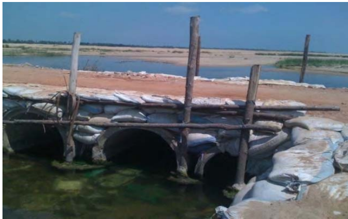
(Photograph of long path laid at Mudivarthipalem)
