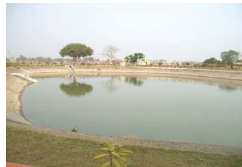
Pond in the WTP area
