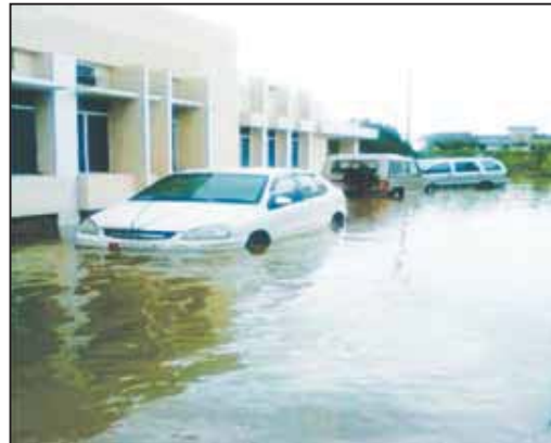
File photo of 132 KV SS building at Kashipur during flood
