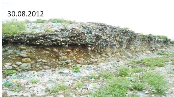
Waste being washed away by flood in Gola river Haldwani (old dumping site)
