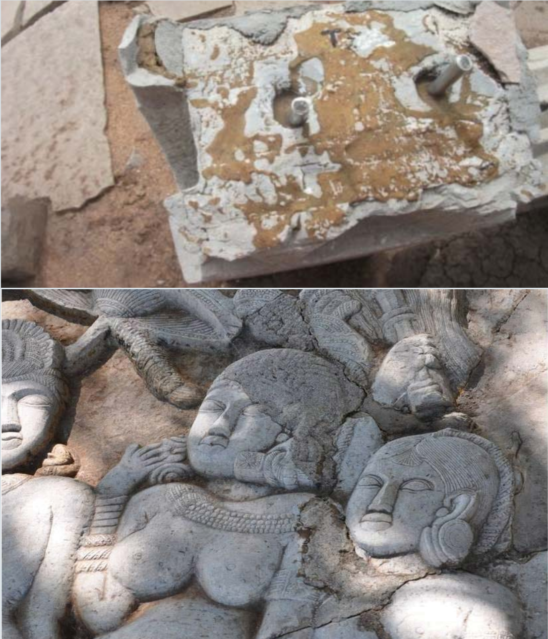
Faulty Repair works at the site
