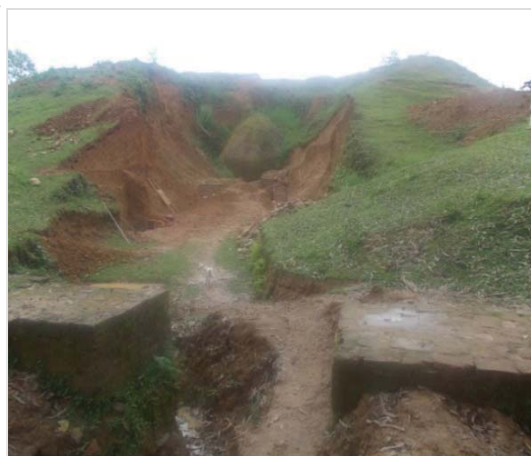
Current view of Excavated Maidam at Charaideo, Sivasagar, Assam as on 10/06/2012
