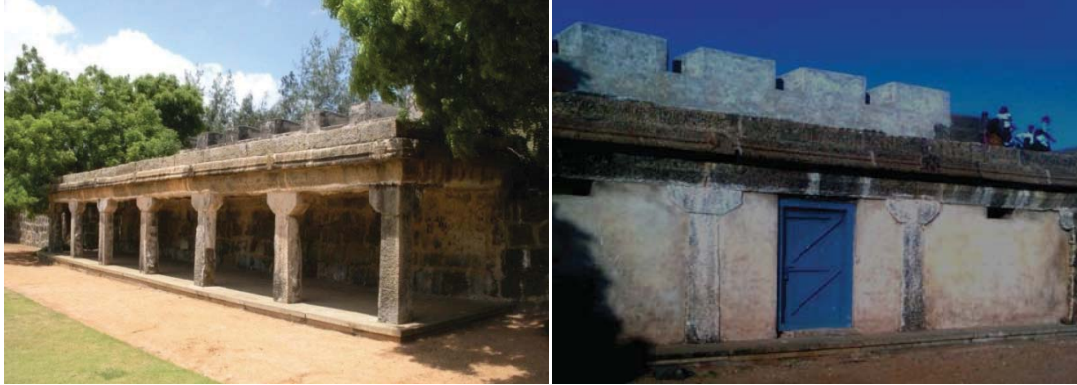
Mandapa's original look and after conversion to store house
