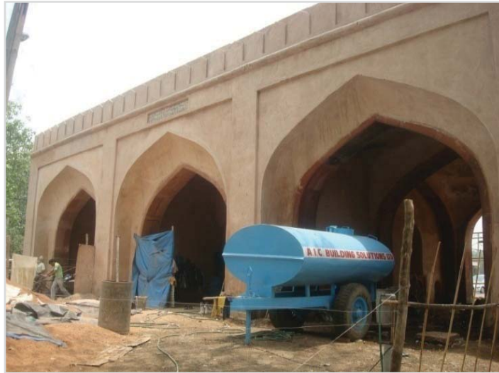
Tripolia Gate after conservation (missing designs)
