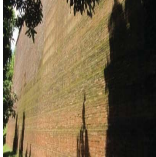
No recess in the reconstructed wall
