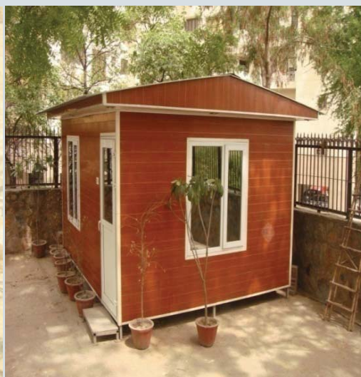
Porta Cabin erected by GVO
