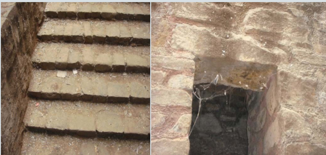
Non maintenance of the monument by the GVO
