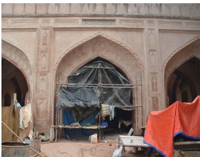
Tripolia Gate before conservation
