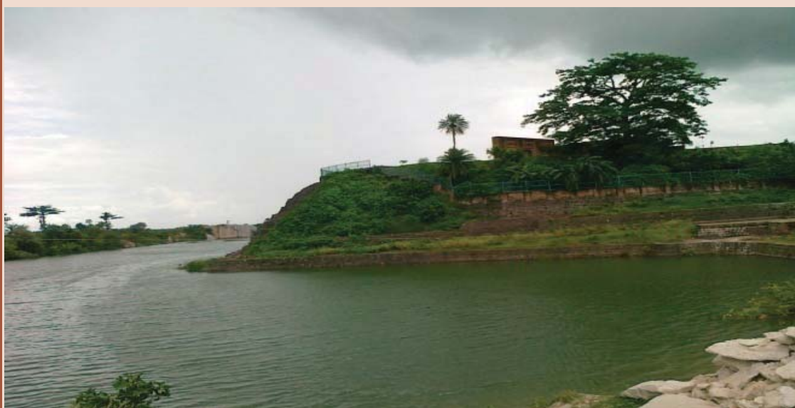
Water logging in and around Baradari Site
