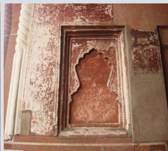
Fading of plaster of Paris in the Mehman Khana
