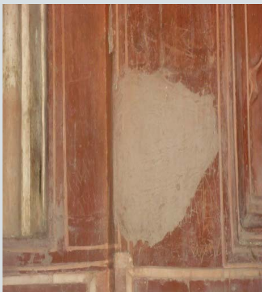
Cement work on wall in the mosque
