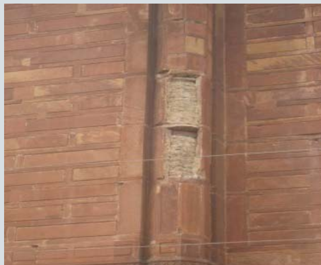
Missing stone and plaster
