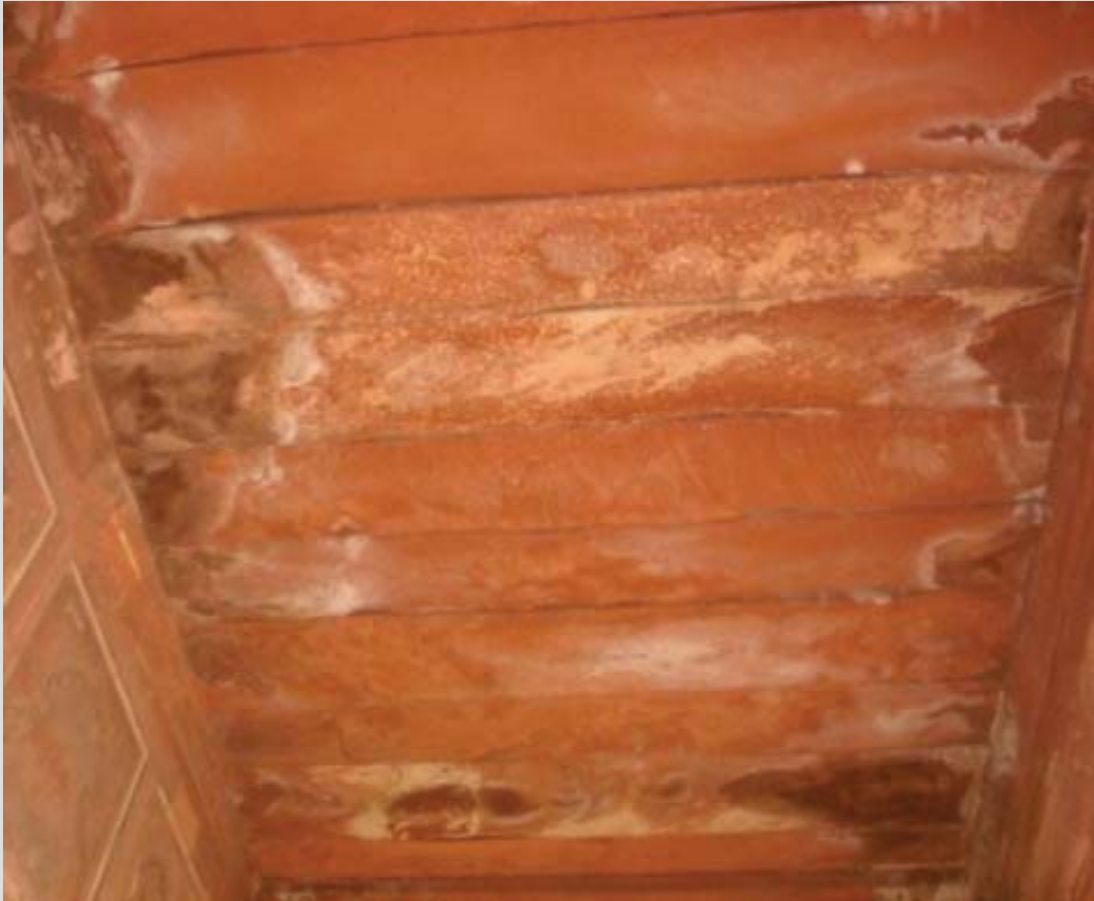
Seepage on the roof
