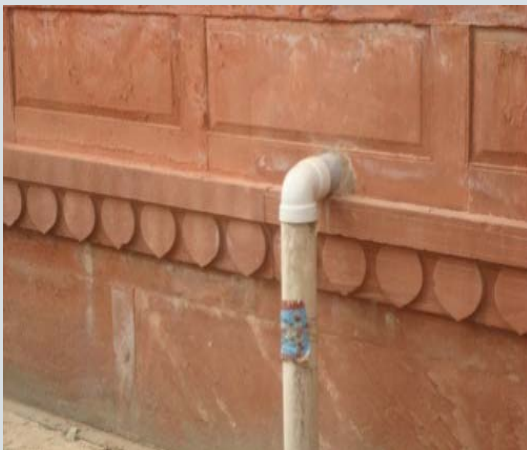
Plastic pipe fixed in the wall
