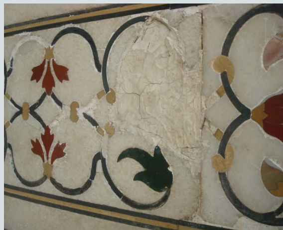
Patch work of the inlay work
