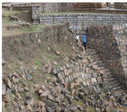
Chinnakavandanur, Sangagiri - Damaged side wall of the lower tank
