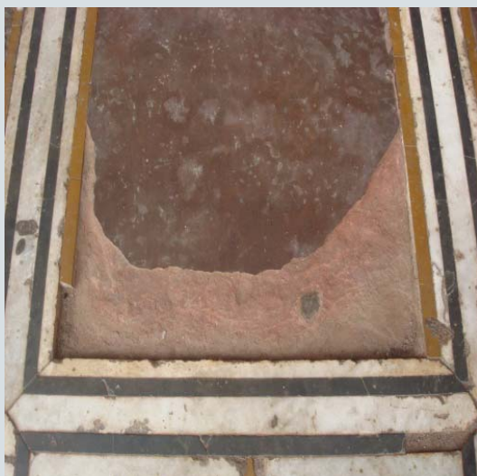
Broken flooring of the mosque
