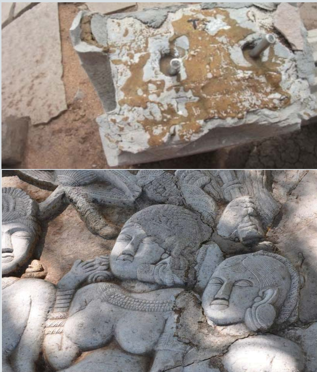
Faulty Repair works at the site
