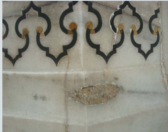
Patch work on the marble design
