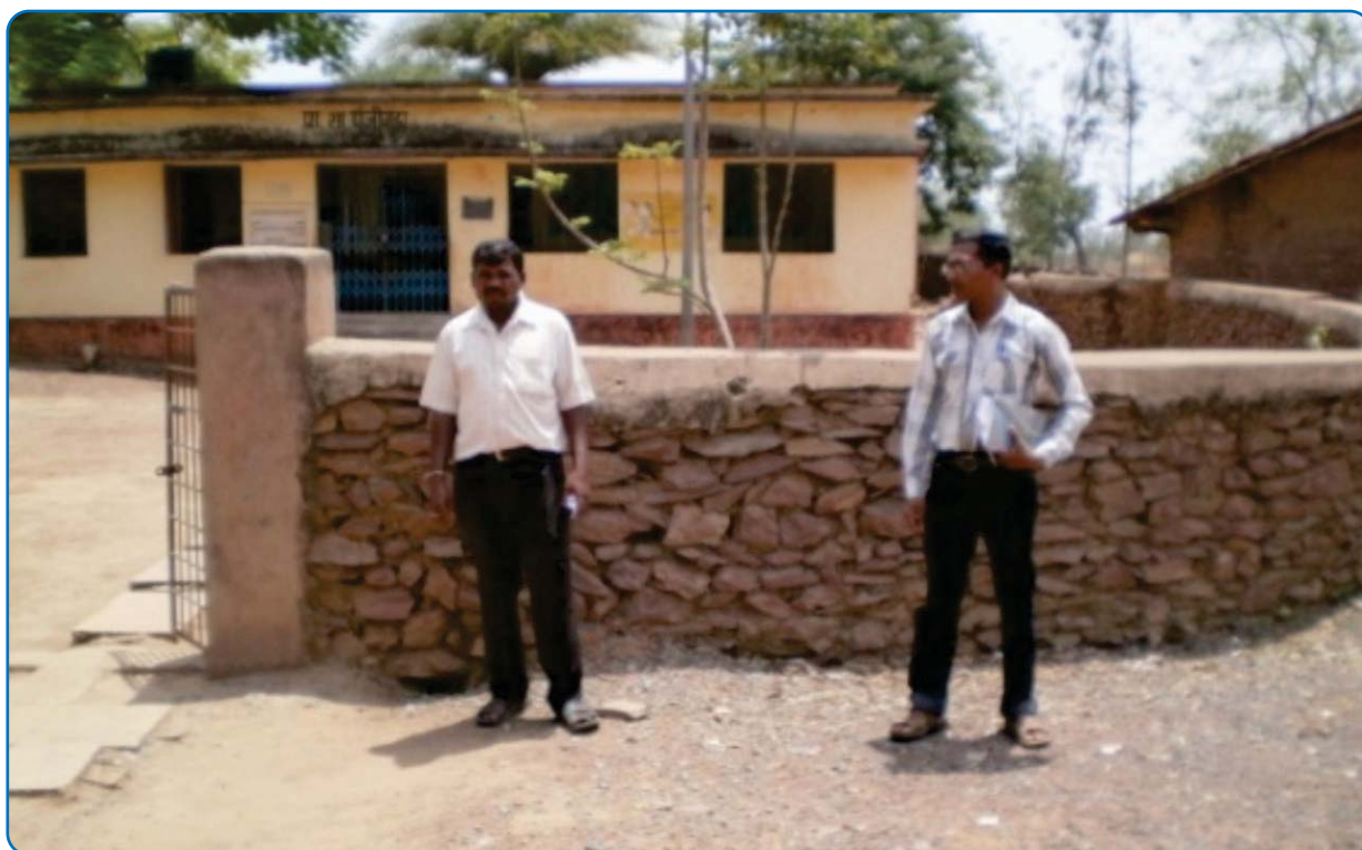
Construction of boundary wall at village bhond, block Bastar, district Bastar, Chhattisgarh
