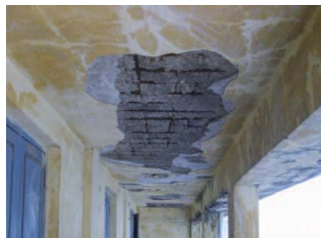
Damaged ceiling of verandha GHSS, Sultanpet
