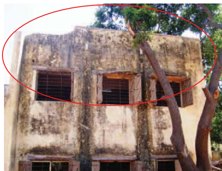
Broken parapet and sunshades in GPS, Muthirapalayam
