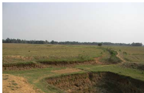
Renovation of Ketuapal Creek
