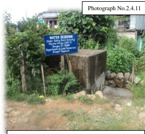
Water Reservoir constructed under EPA-Pherima village
