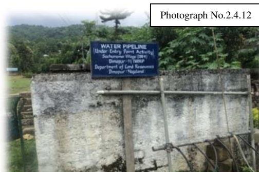
Water pipeline constructed under EPA Sochunuma village
