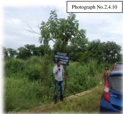
Culvert constructed under EPA Razaphe village
